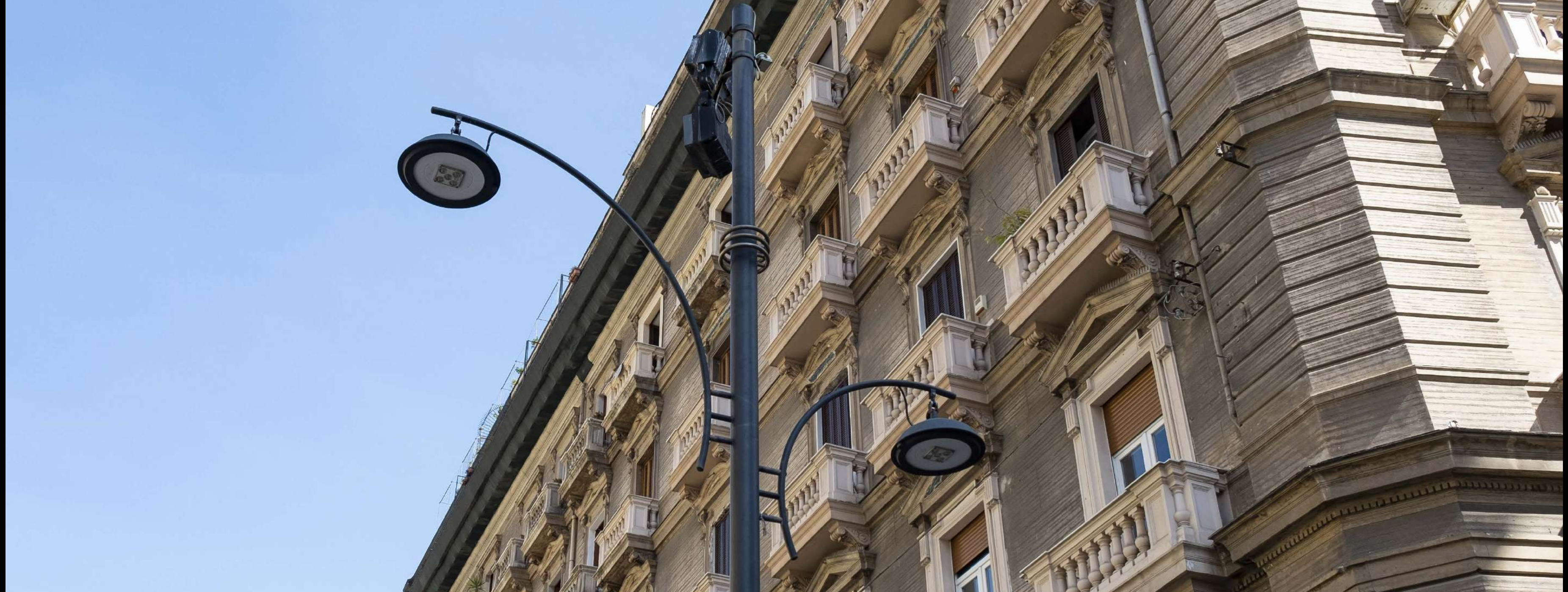
Cree Lighting street luminaires on the central streets of Naples | Product pictured: Urban Series
